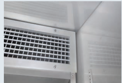
Adjustable Double Deflection Grill for Optimum Airflow
